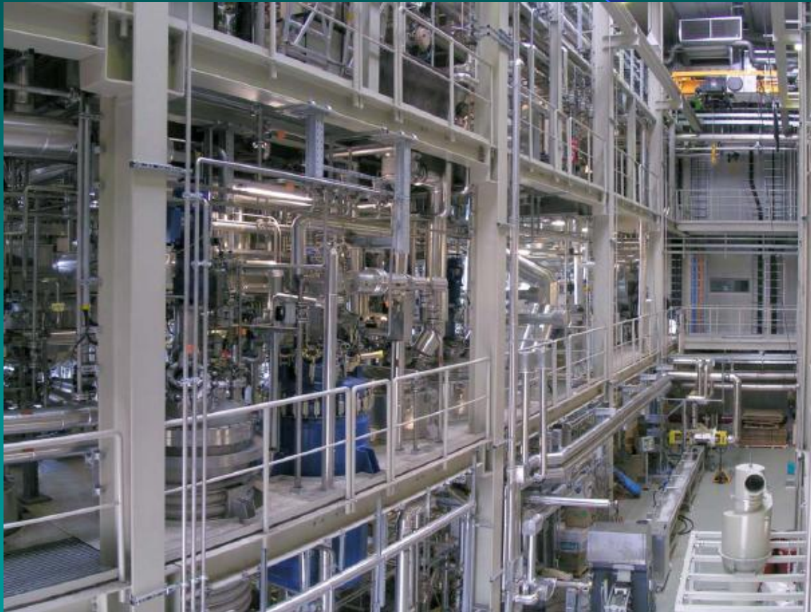
Polymerization Pilot Plant
